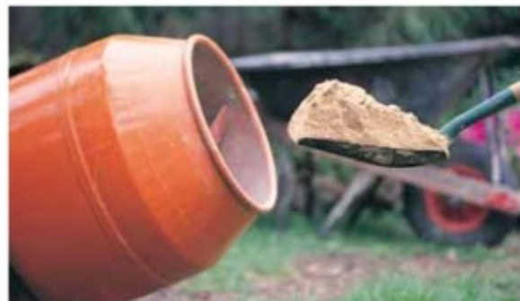
Figure 22 Mortar Mixing (Sand Addition)
