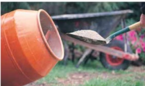
Figure 21 Mortar Mixing (Cement Addition)
